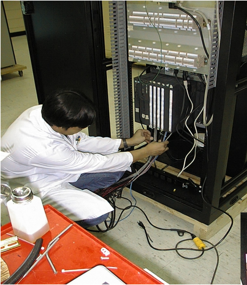
Wiring and Calibrating PLC
