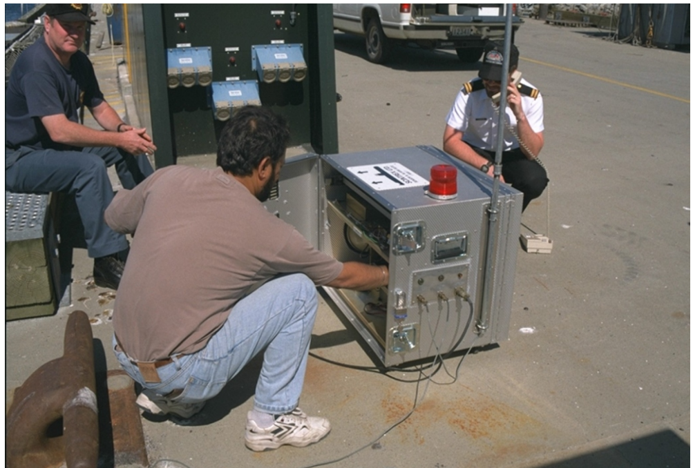
Installing System at CFB Nanoose
