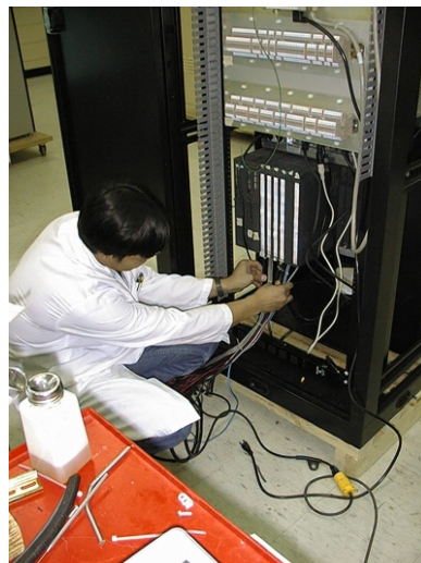
Wiring and calibrating PLC modules
